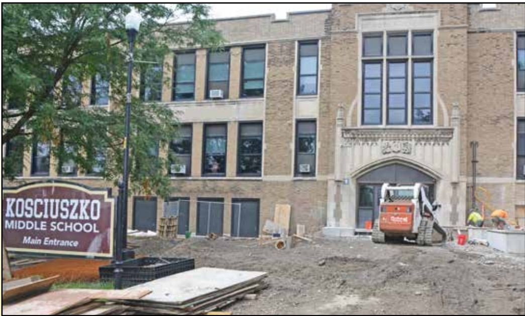
Kosciuszko Middle School had its windows replaced thanks to a past federal covid pandemic relief grant. A number of other district buildings underwent repairs as well from the funding. But now, the federal government is clawing back a promised $7.2 million in that funding. File photo
