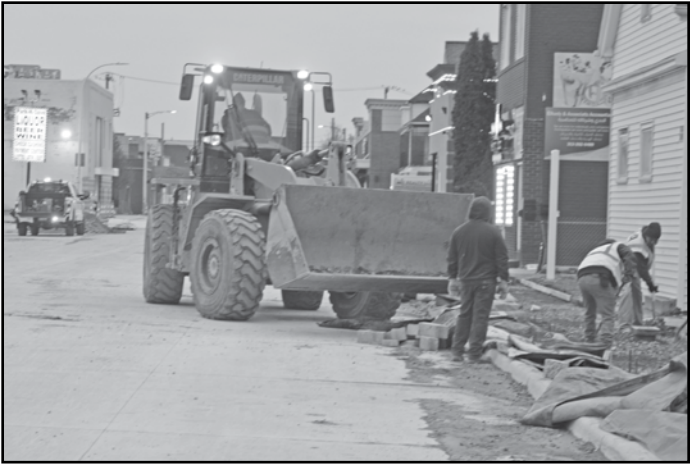
The last phase of repaving Caniff from Jos. Campau to Conant could only be partly done. Reconstruction of the street will begin again in spring.
