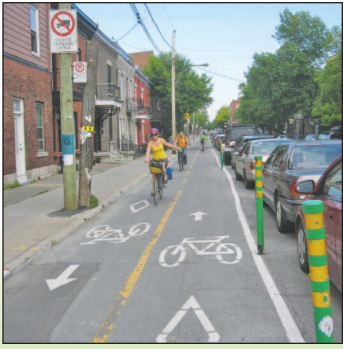
One way to reduce speeding drivers is to create bike lanes, forcing drivers to slow down and share road space.
